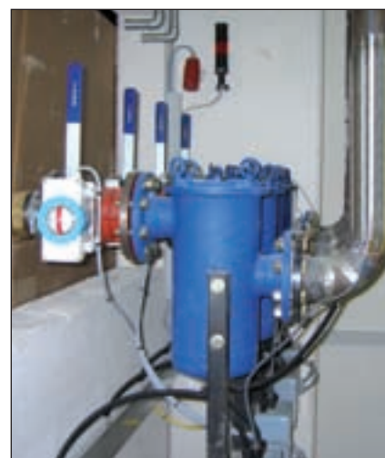
Filling filter for bulk container system
